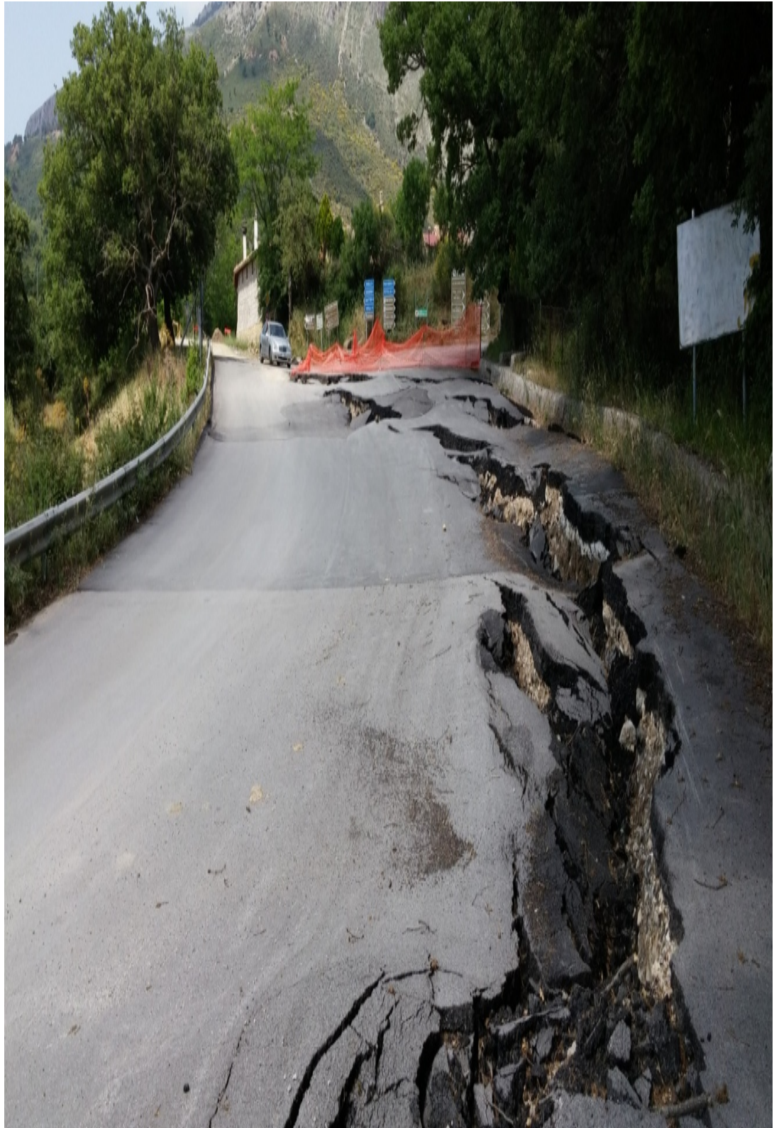
Plate 2.5: Block cracking
