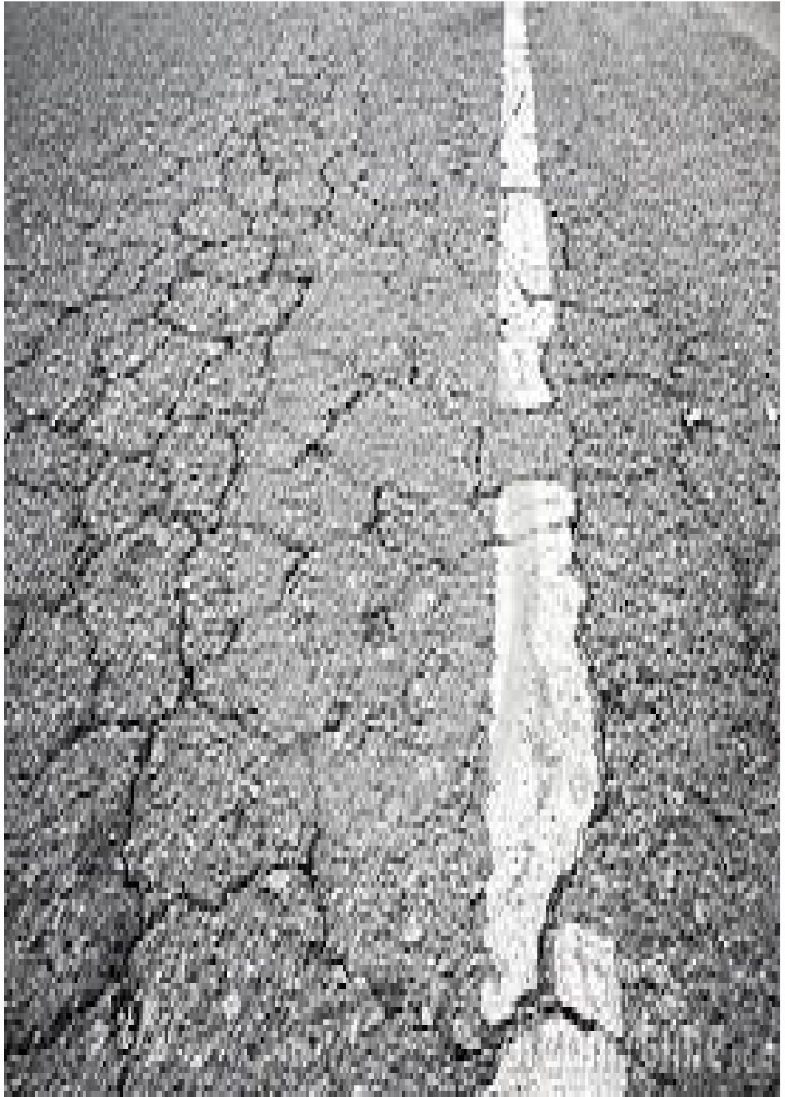
Plate 2.1: Alligator cracking.
