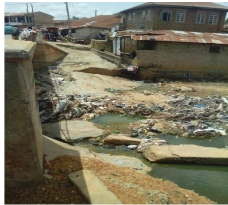
Plate 7: Emir bridge, ASA RIVER [AS5/SW5]
