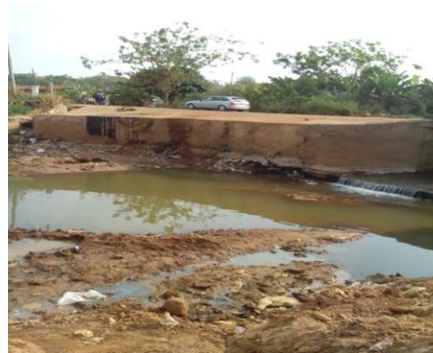
Plate 4. Cocacola road mixing point [FB/SW3]
