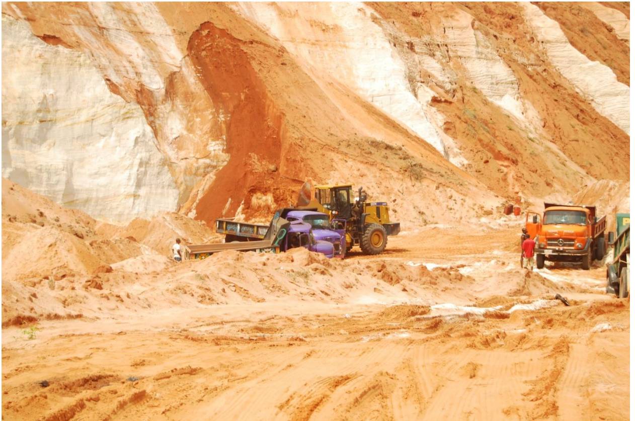
Plate 4.8: Tippers waiting to be loaded by excavators at Abudu
