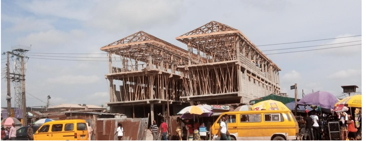
Fig. 4.29: An on-going shopping complex in Alimosho LGA
