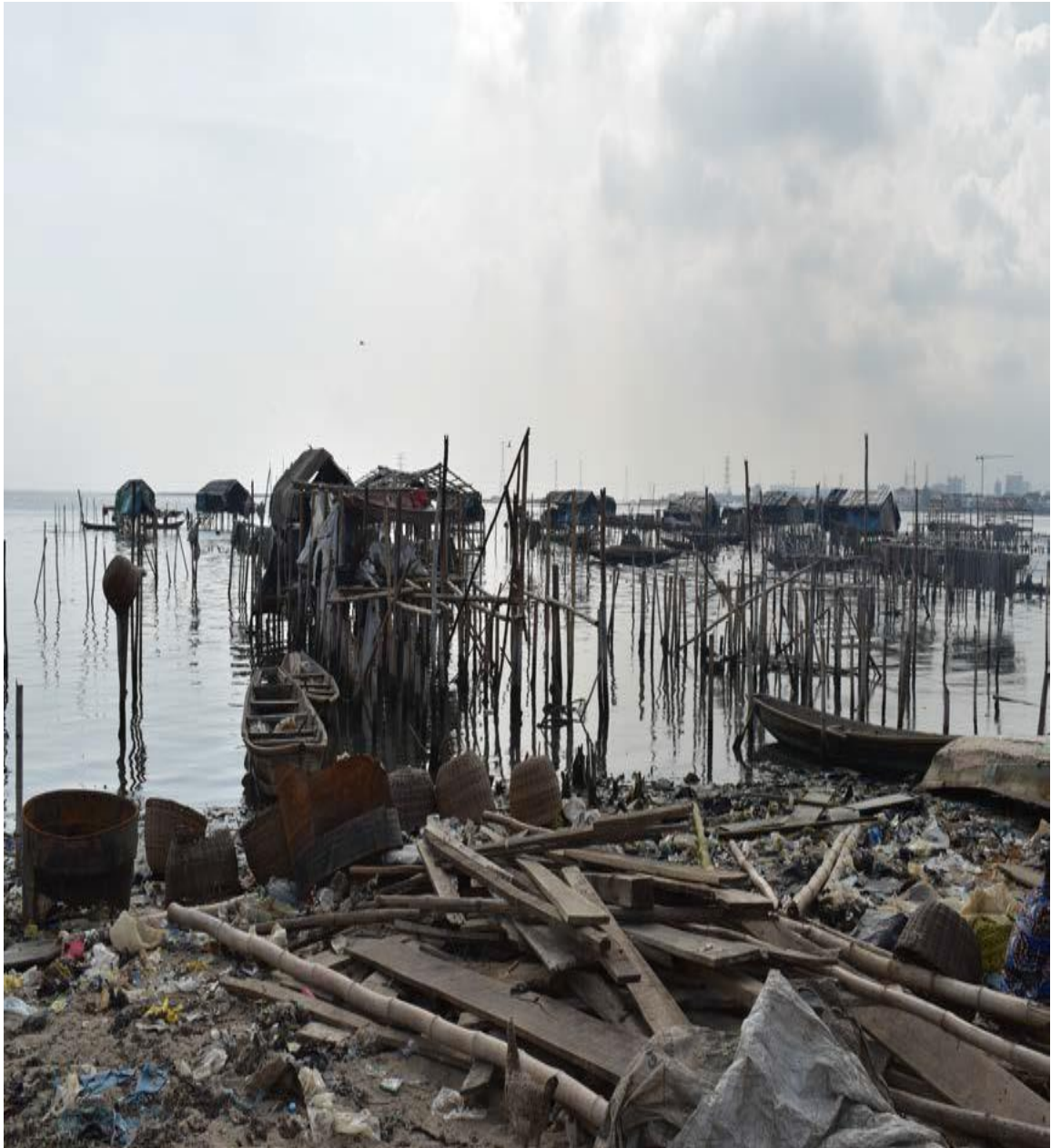
Fig. 4.7: Image of the Rubbles of Demolished Ilubirin Community
