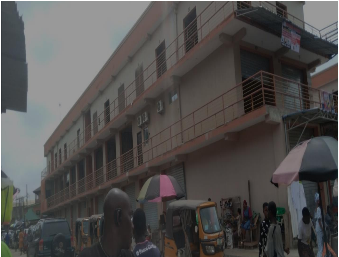
Fig. 4.14: An Image of a Massive Shopping Complex in Oshodi
