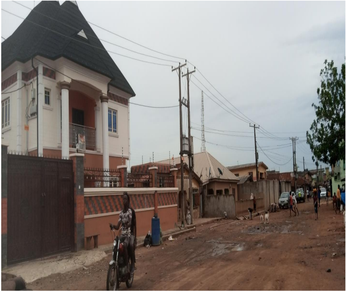
Fig. 4.16: A pictorial evidence of residential gentrification.
