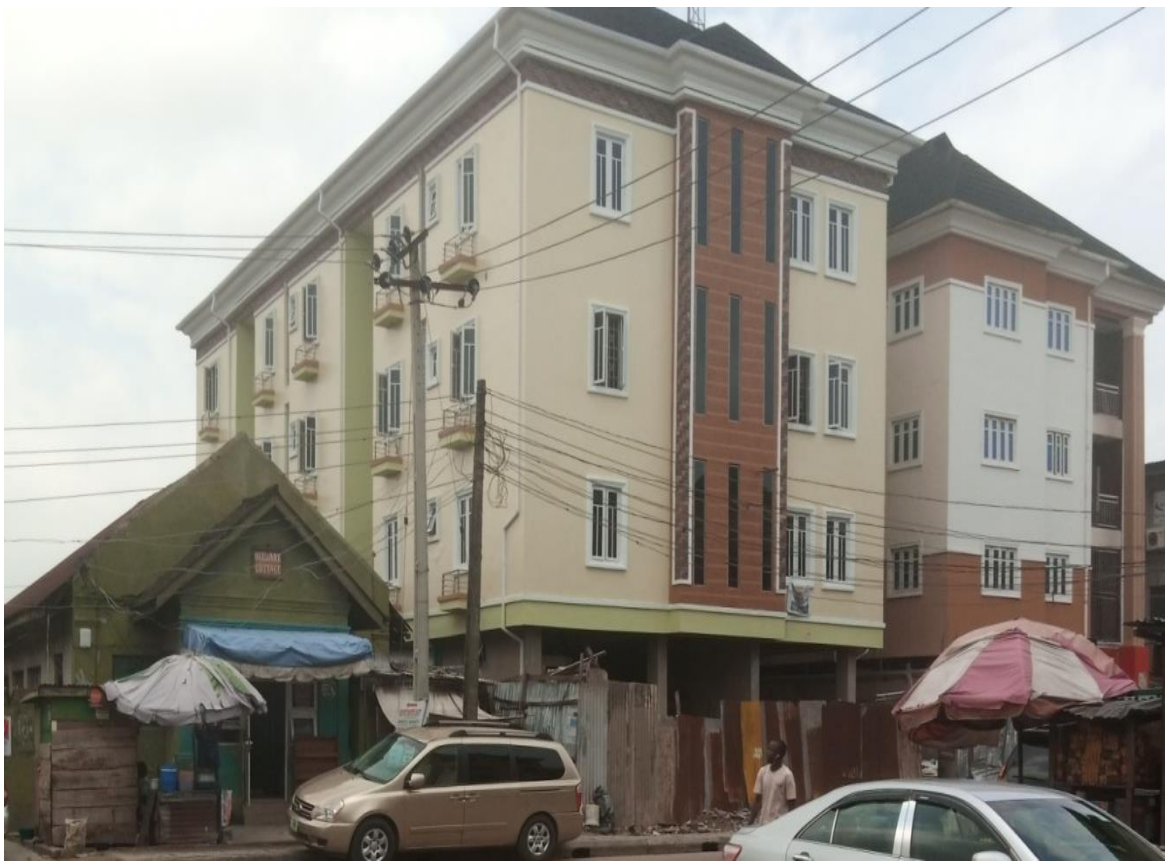
Fig. 4.23: Some On-going and newly re-built High Buildings in the Lagos Mainland
