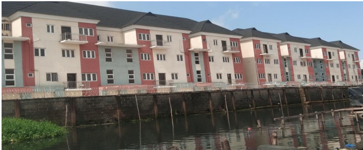
Fig. 4.32: Images of the Lagoon View Estate built in the heart of Makoko slum
