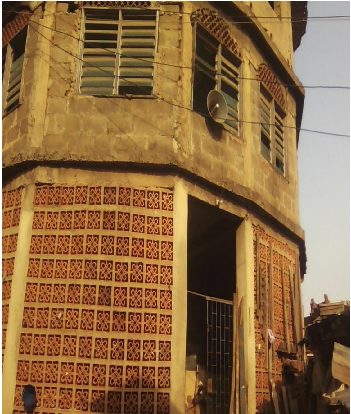
Plate :4.5: The modern structure and front view of Onisiriniyan Mosque, Oritamerin area, Ibadan; the first Mosque with roofing sheet and Islamic Centre in Ibadan
