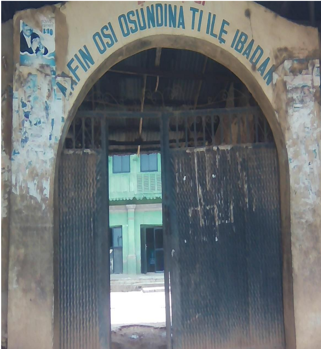
Plate 4.3: The main entrance gate to Osundina Compound, Ibadan. Source: Fieldwork 2017
