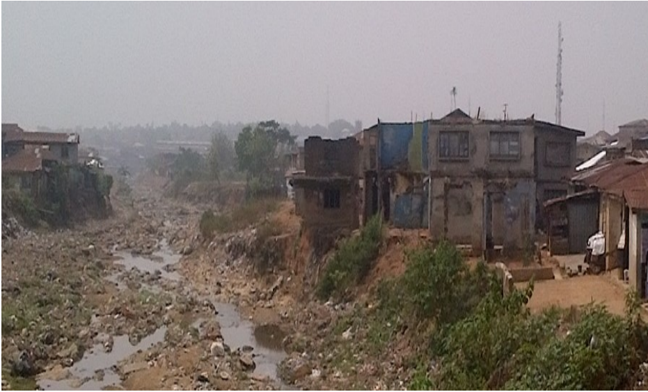
Plate 4.4: A Devastated High-Rise Building along Kudeti Stream, Ibadan
