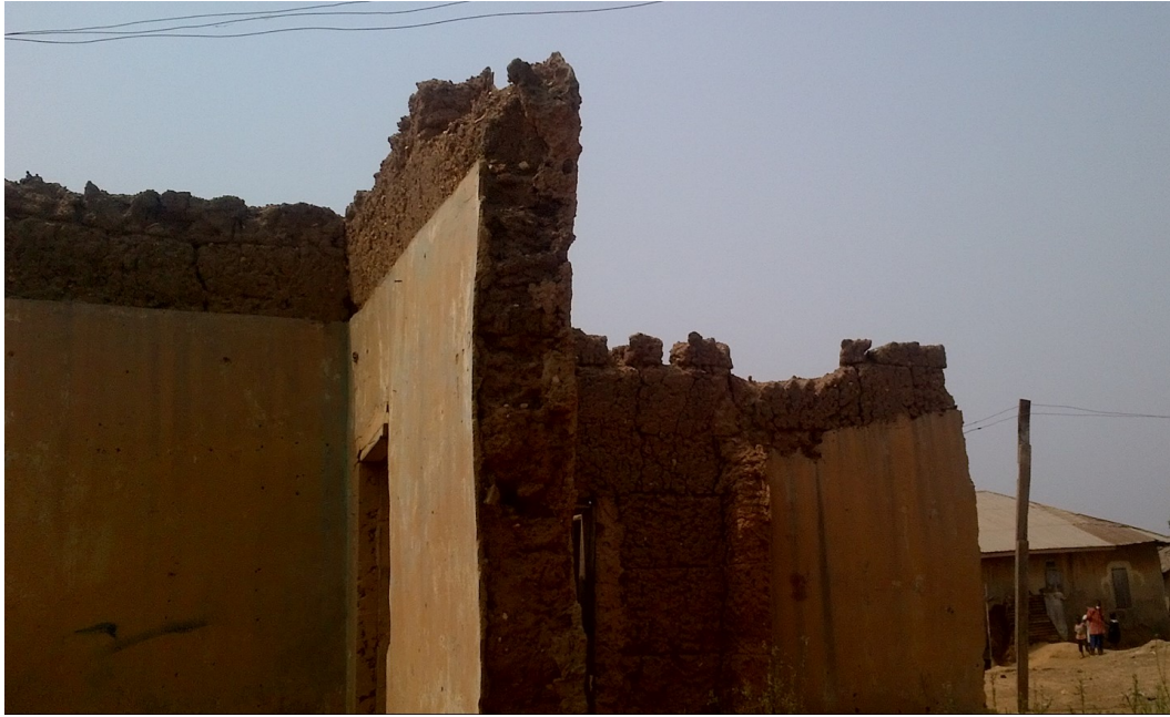
Plate 4.14: Windstorm Devastated Mud Building at Morgana Compound, Idiarere, Ibadan
