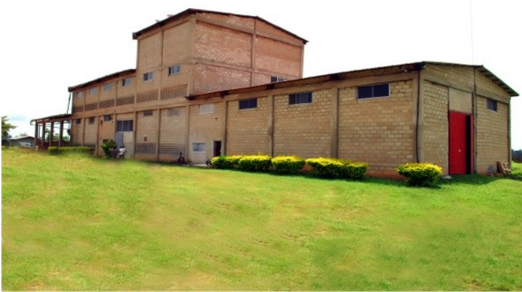
Matna Foods factory building
