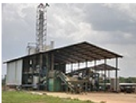
The processing plant
