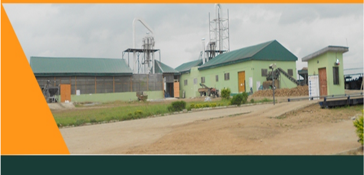
Psaltry company factory building
