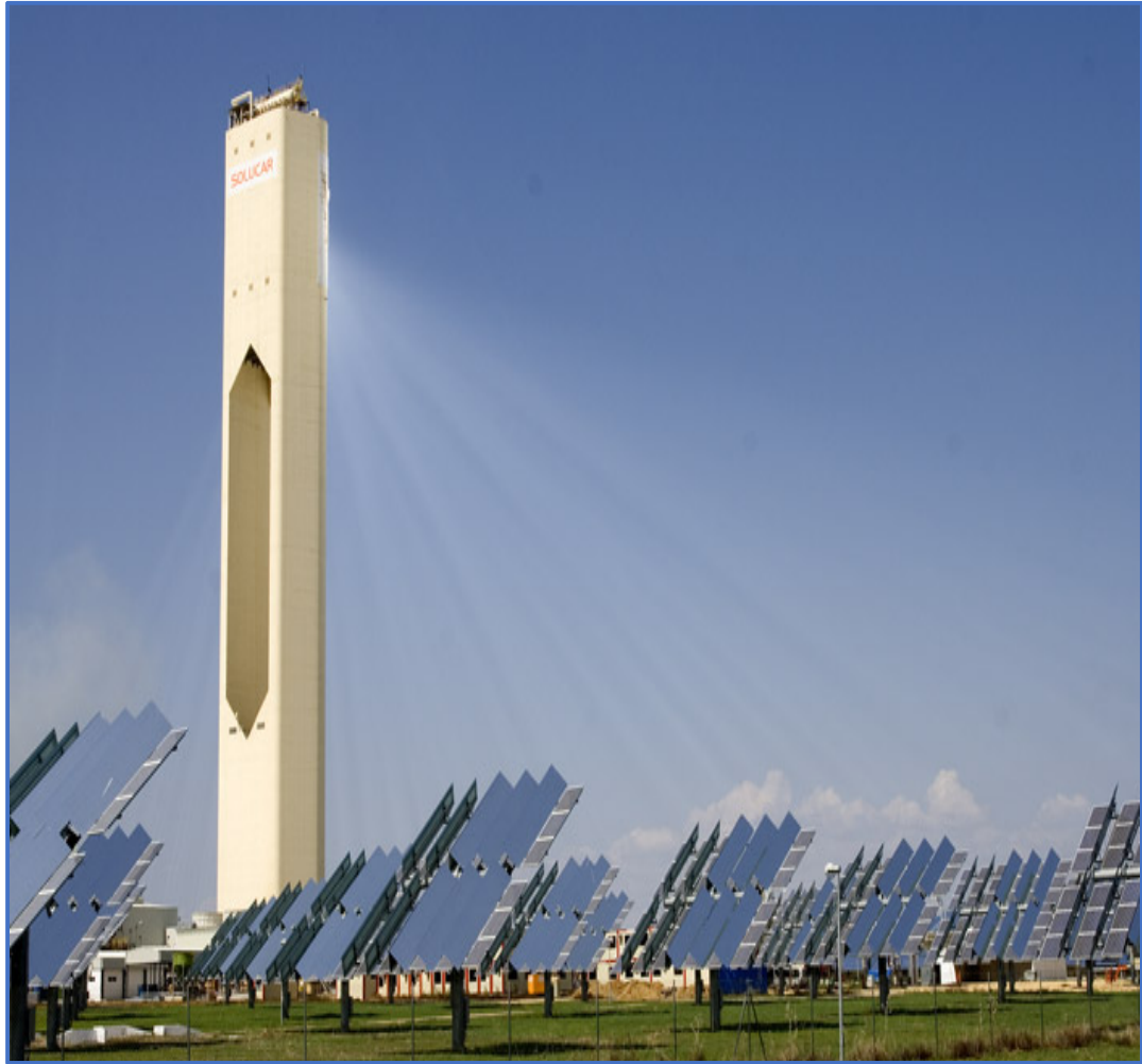
Plate 2.1: Pictorial Model of a CSP Central Receiver System (Source: U.S. Dept of Energy, 2013).
